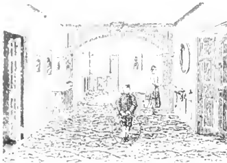
HALLWAY OF THE OLD MANSION, 1663.
